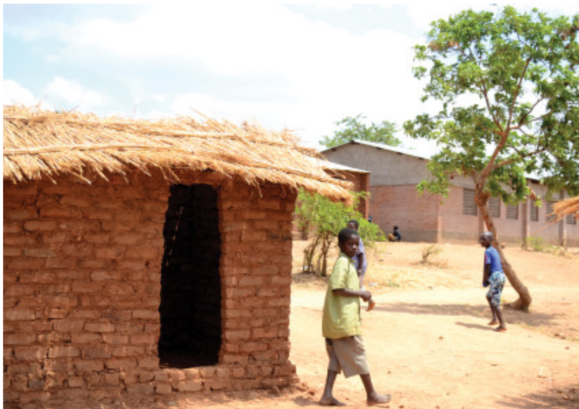
Chigumba new classrooms and existing toilets
